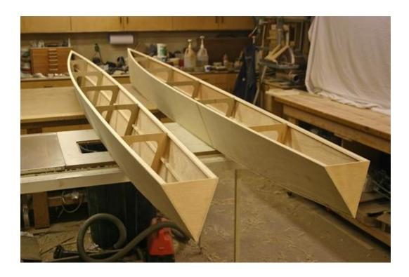
11) Fair out the sheer stringer and frames. Check the deck for flatness with a straight scrap of wood. Fit the two layers of 1/2" plywood for the beam attachment. The bottom layer fits under the sheer stringer, the top flush with the deck. Epoxy in place. Glue the 1 1/2" x 2 1/2" x 2 1/2" block under the beam attachment. Fit the 1/4" plywood frames that reinforce the beam attachment. Screw in place with epoxy, and bond to the hull with an epoxy radius and glass tape.
